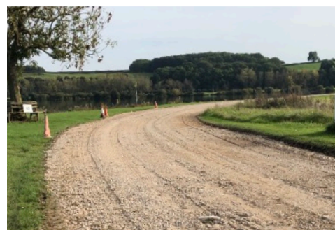
Above: track graded
